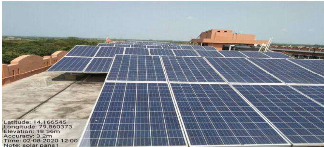
300 KW Solar Panels on the roof
